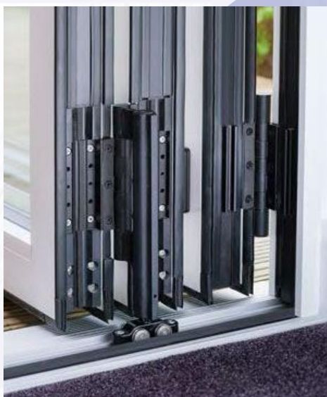
3D Detailed View Bottom Frame with hinges
