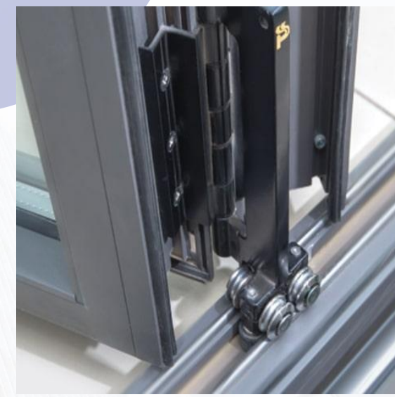
3D Detailed View Non Thermal Break Window
